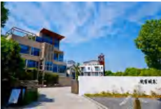
Figure 45: Main Village Entrance
