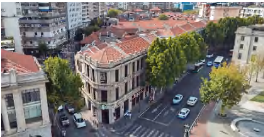
Figure 96: Bird's View of Baoyuanli
