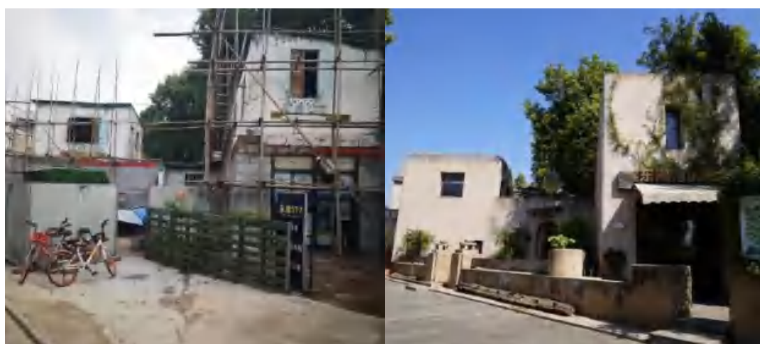
Figure 43 : Pompei Restaurant Before and After Renovation
