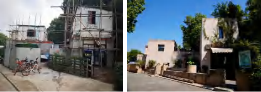
Figure 52: Pompei Restaurant Before and After the Renovation
