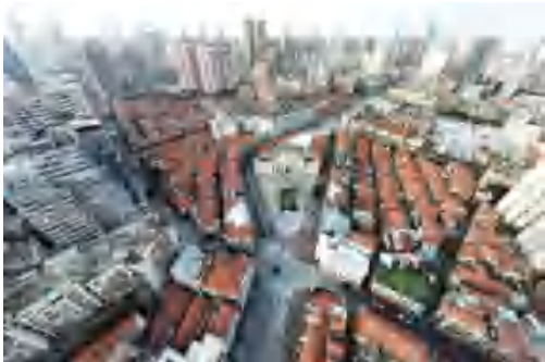
Figure 4: Renovation of Zhongshan Avenue, Wuhan
