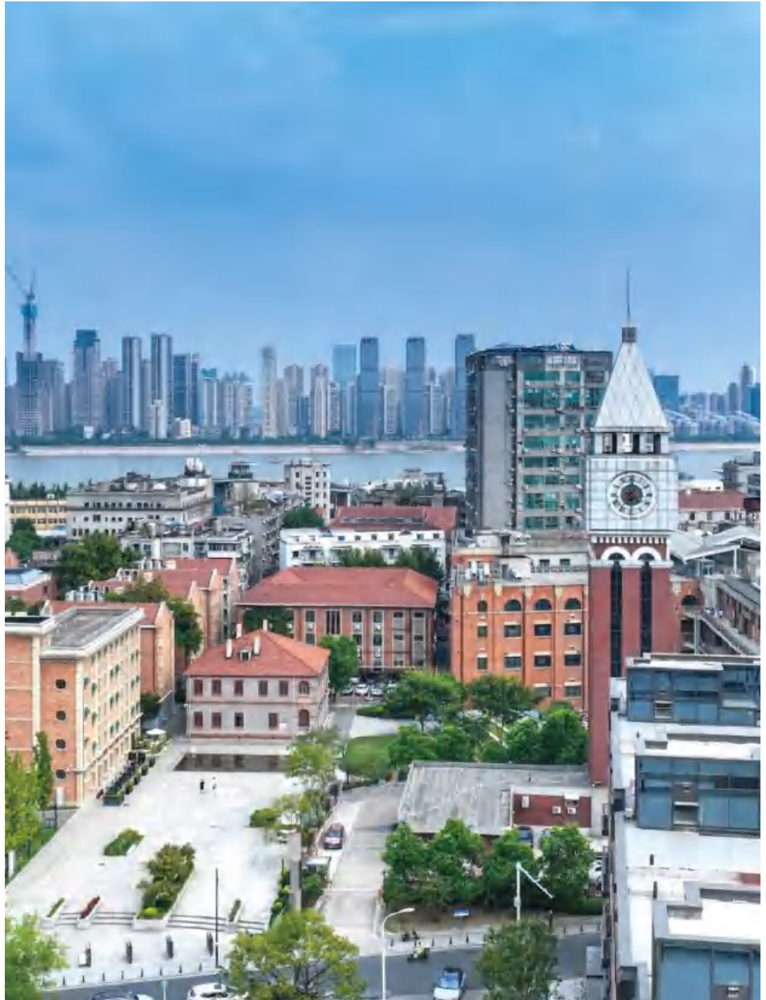
Figure 73: Bird's View of Pinghe Workshop
